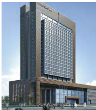
Commercial Building Building area: 65,000 m 2 Cold storage capacity: 3,852RTh
