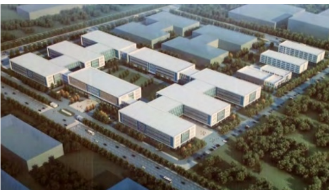
Industrial Park Building area: 197,781 m 2 Cold storage capacity: 16,380RTh
