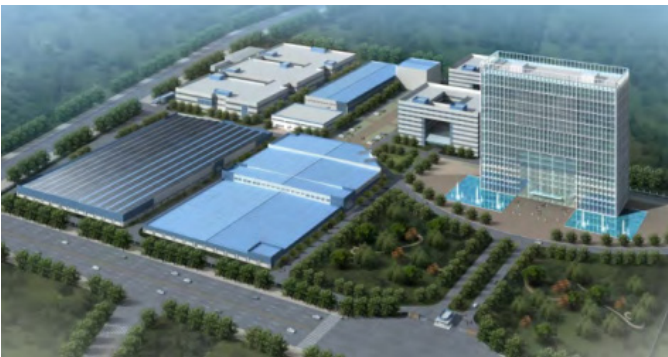
Industrial Park Building area: 300,000 m 2 Cold storage capacity: 20,930RTh
